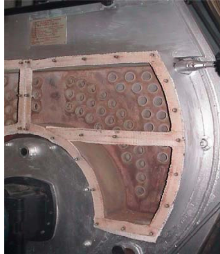
Post Fitch Installation 48 hours
